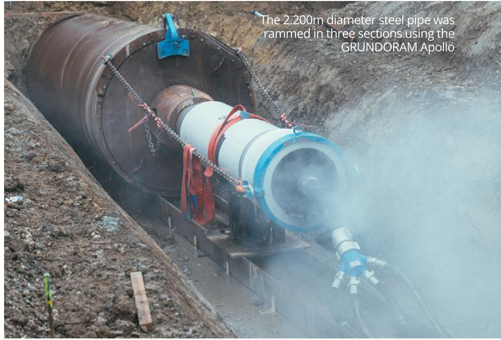
Pipe ramming under the motorway was carried out while traffic was moving, with the sewer being installed with 4.20m upper edge - without causing any damage to the motorway
